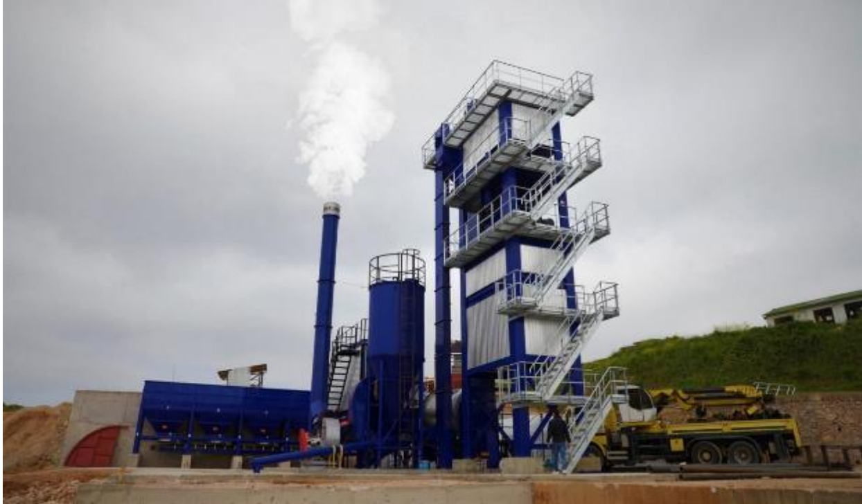
Image 6: Bandırma Municipality Asphalt Plant
